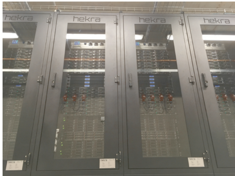
Figure 9.1: Cooling cabinets with a HPC cluster in one of the server rooms at MPI-DS. Each cabinet has a control and monitoring unit, is built in a modular way so that it can be moved, and can be customized to cool up to 36 kW if necessary.
