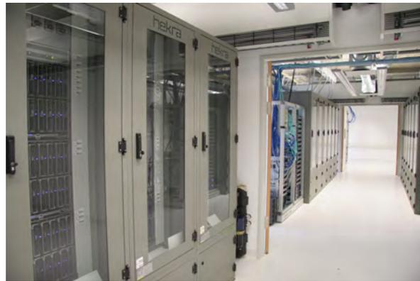
Cooling cabinets with HPC clusters in the main server room of the department of Nonlinear Dynamics. Open racks for infrastructure servers in the front. The cabinets have a dedicated control and monitoring unit, are built in a modular fashion so that they can easily be moved, and can be customized to cool up to 36 kW.
